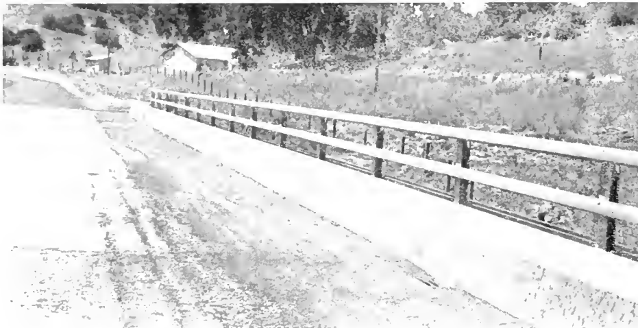
Use of railroad rail railing on Poso Creek Bridge
